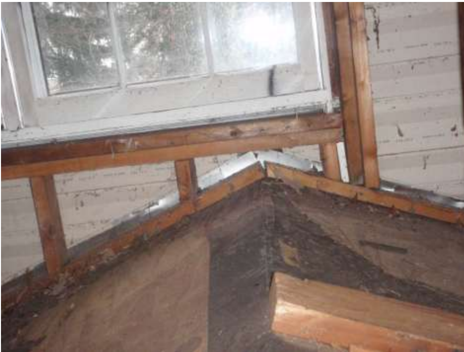
Leakage from the uninsulated wall in the living room attic, adjacent to sunroom (above), is visible below as heat escaping (red).
